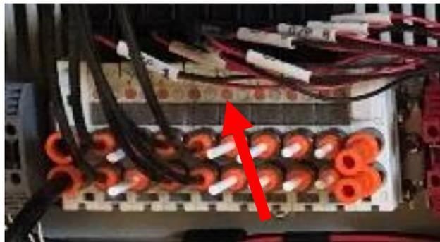
From left to right, the first valve is the robot gripper followed by an unused valve, the rotating grip station nearest to the pump (S2), and the other rotating grip station nearest to the tray (S1).
