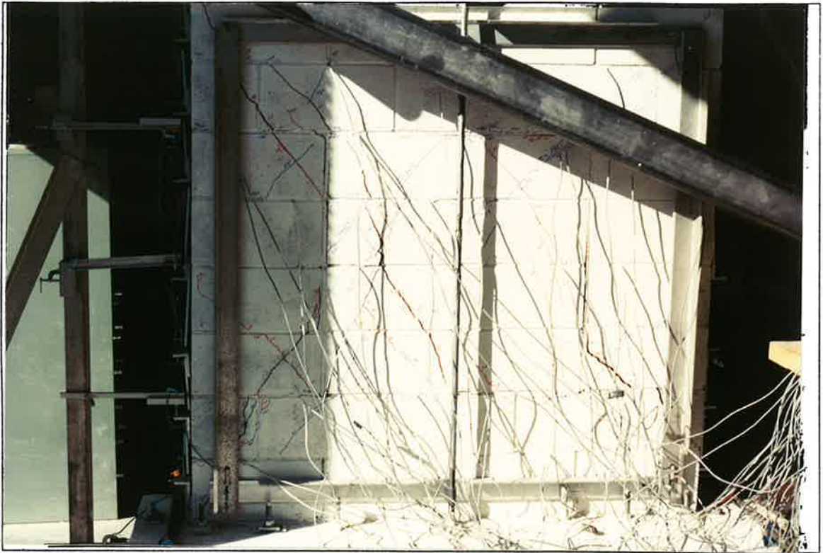
Photo B.13 Slitted Wall South Face At 245 kN (55 Kips) Lateral Load
